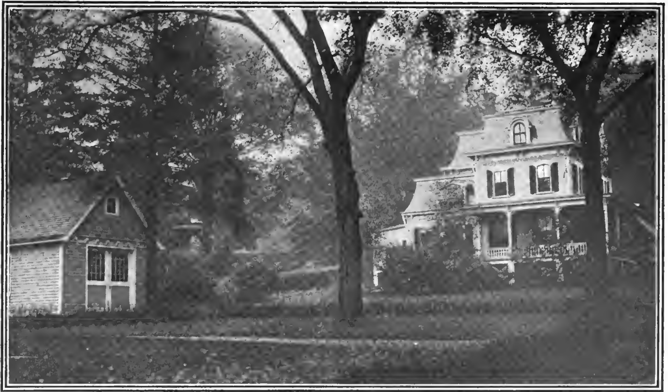
Wooden building used to house the car of one suburbanite who has business in New York
